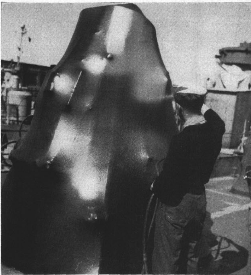
STRIPPABLE FILM —another plastic—is sprayed over the gun mount of a ship being mothballed. This method was widely used and saved millions of dollars.
