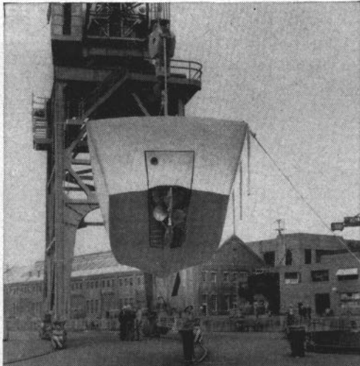
COMPLETED boat, with its engine and propeller unit installed, is taken to the water on a giant crane at
