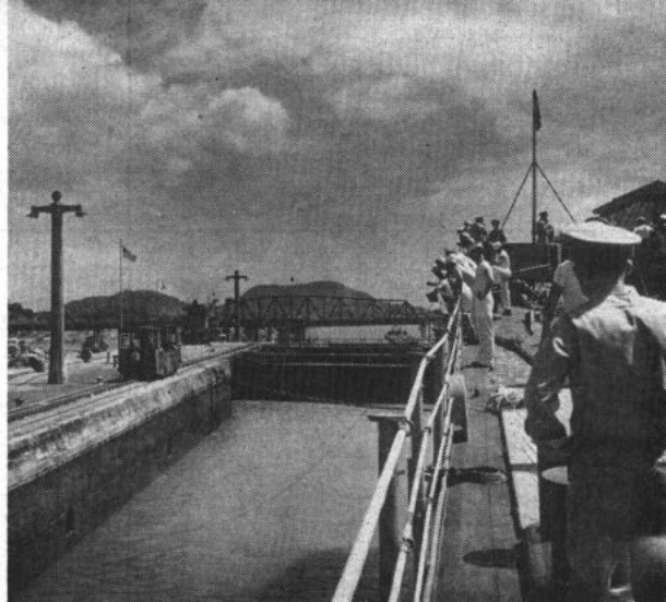
6—TWO LOCKS at Miraflores return ship to sea level. Chains across locks prevent damage through ramming.
