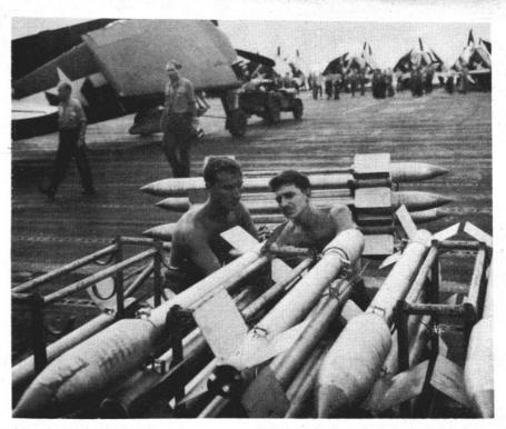
DEADLY BUT DELICATE, rockets are carefully checked and rechecked by these trained Navy ordnancemen before their installation aboard carrier-based planes.
