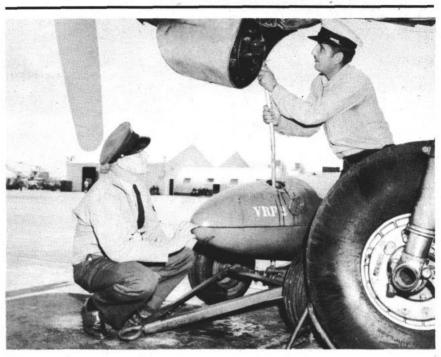
OIL BOWSER is name of contraption being used by its designers at NAS, San Diego, to drain oil safely from aircraft engine. Device came from the junk pile.
