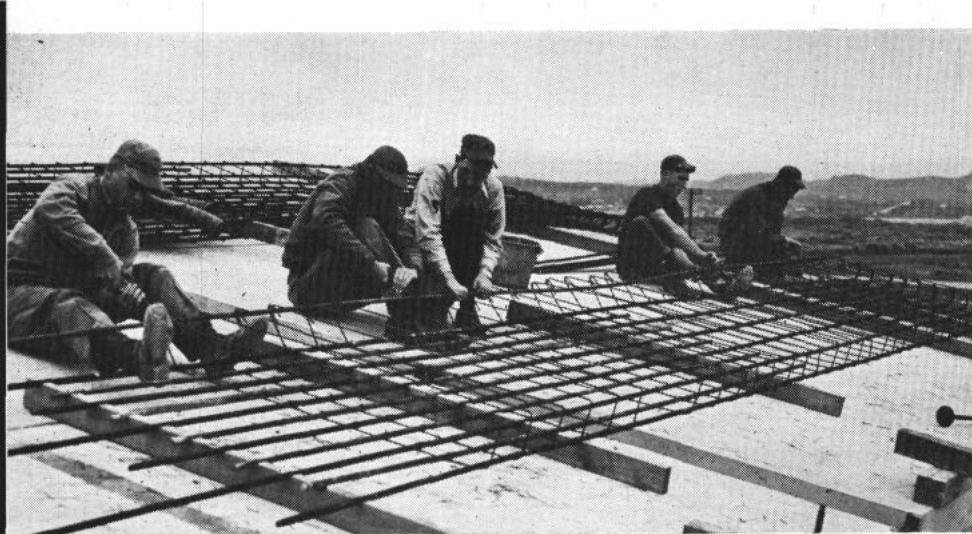
STEELING THE SHOW —Steel Workers assemble reinforcement for concrete.
