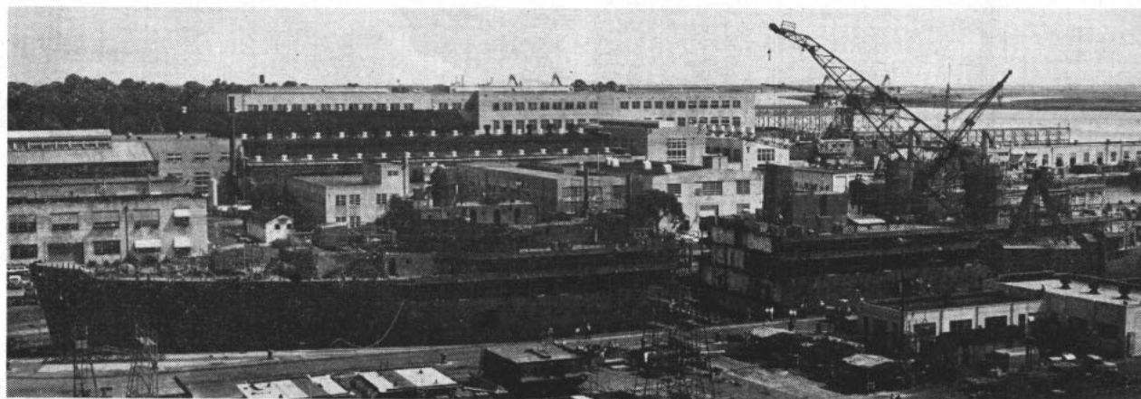
MID-RIF — USS Proteus (AS 19) lies in drydock at Charleston, split in half to add new midsection that will equip her with special shops and gear to serve as a Fleet tender to the Navy's first squadron of nuclear submarines.
