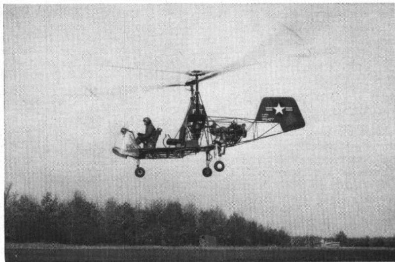
THRIFTY WHIRLYBIRD —The new engine, similar to one used on turbo-jet planes, will enable 'copter to fly on kerosene instead of high octane gas.
