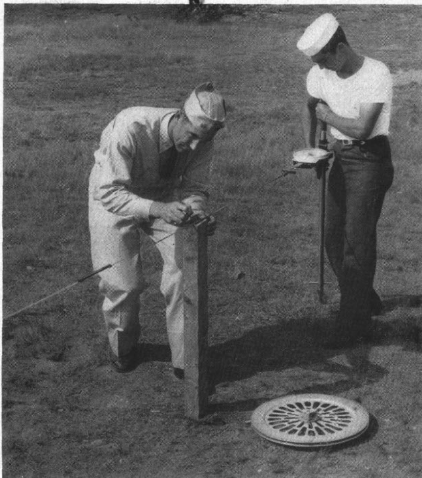
FIRST STEP in triangulating is to measure off a precise base line (above). Teams like this one move about by truck, use only most modern equipment.
