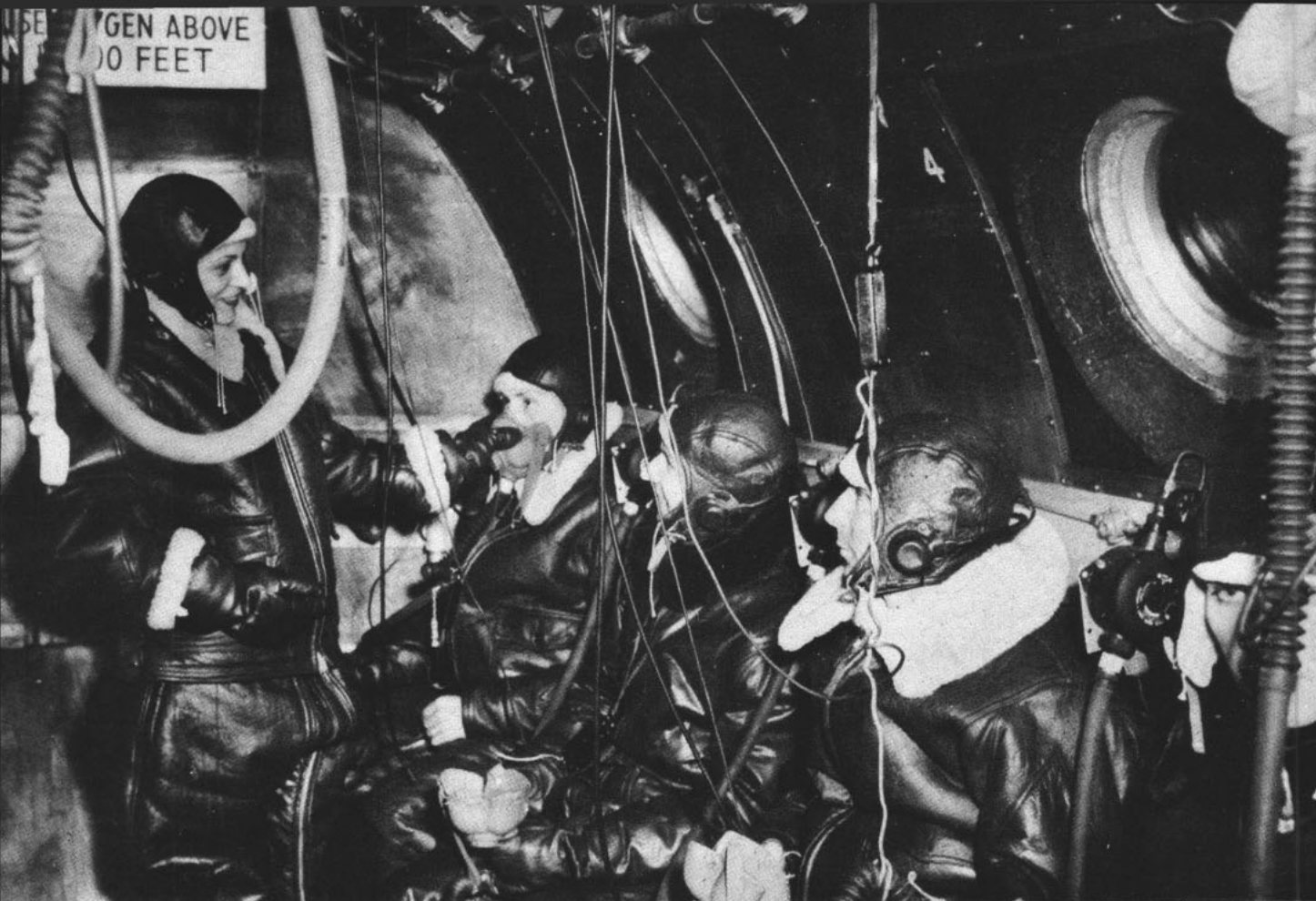
LOW PRESSURE chamber at NAS Pensacola takes men many miles above the earth by simulating high altitude conditions.
