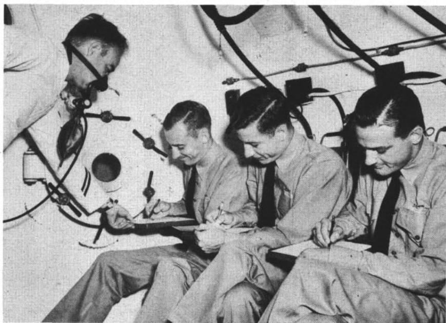
PILOTS at 18,000 feet in simulated altitude think they're doing fine on tests. Because of lack of oxygen, they actually are failing simple problems.
