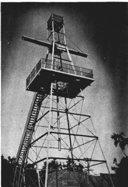
LIVE fuzes mounted in bombs receive drop-tests daily from 75-foot drop-tower situated at Naval Ordnance Lab.
