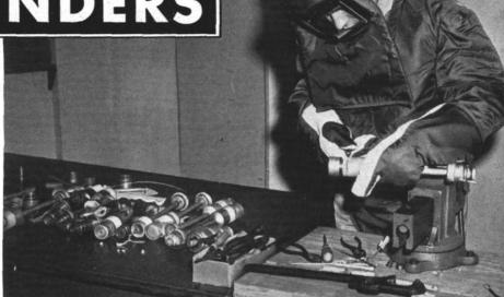
PROTECTION suit of 78 layers of nylon and mask containing viewing part of shatterproof glass are worn by man stripping fuze from the arming pin.
