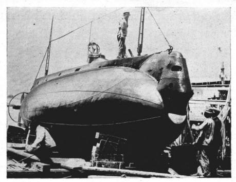
OUR FIRST sub was the Holland, built in 1898 by John P. Holland. She displaced 74 tons, was 55 feet long, and had one deck tube for 18-inch Whitehead torpedo.
