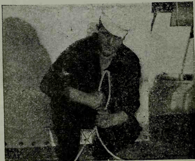
FIG. 47-5—The correct way to take a kink out of wire rope, second step.
