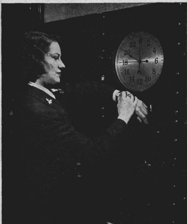
BASIC SIDEREAL Clock (right) measures time between star sights. Punctual Wave at left needn't be more than a few thousandths of a second late after checking her watch with the Observatory's super-accurate transmitting clock.
