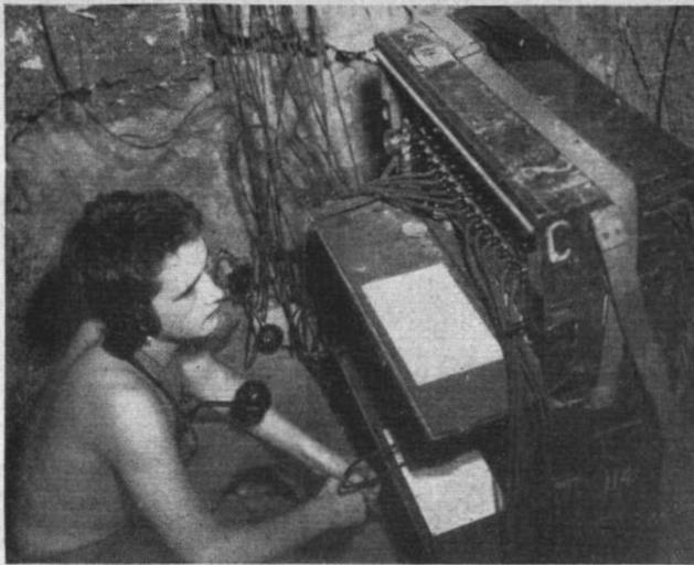
*THE FUNKHOLE ON GUADALCANAL was the sand-bagged communications center. The portable switchboard could be moved at a moment's notice.*
