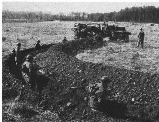
DIG THIS—Mechanical ditch-digger being tested by the Army will provide rapid protection for troops.
