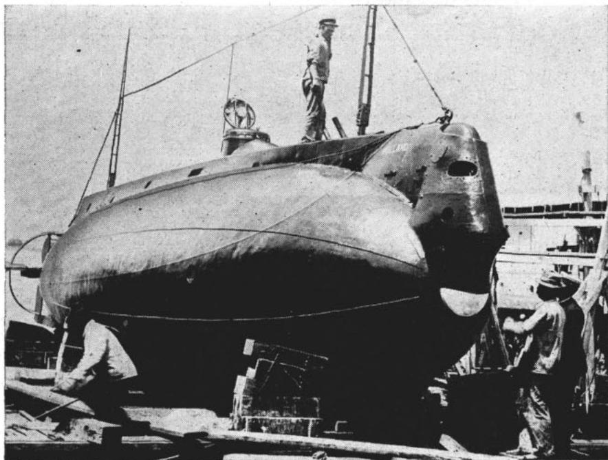
**OUR FIRST** sub was the *Holland*, built in 1898 by John P. Holland. She displaced 74 tons, was 55 feet long, and had one deck tube for 18-inch Whitehead torpedo.
