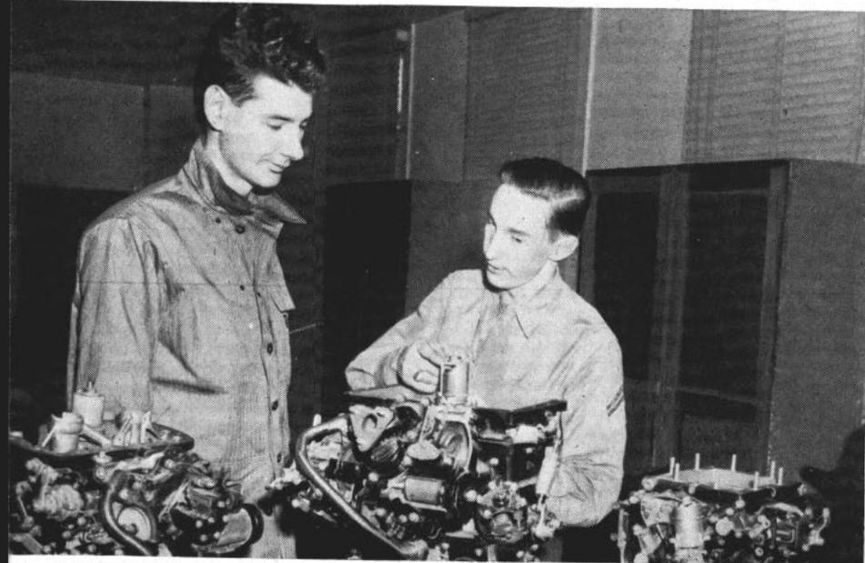
INSTRUCTION on the carburetion system, maintenance and repair of engines are part of the program during which Reservists renew their airplane savvy.
