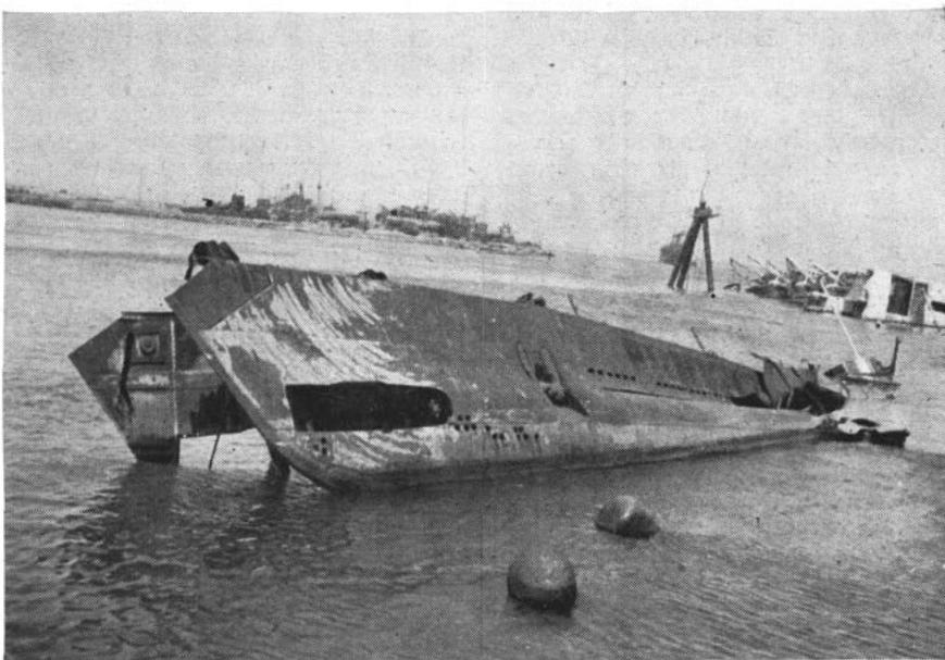
**SUNKEN SUB**, ships block channel at Bizerte. These important waters were cleared by demolitions which sank whole ships beneath channel's sandy floor.
