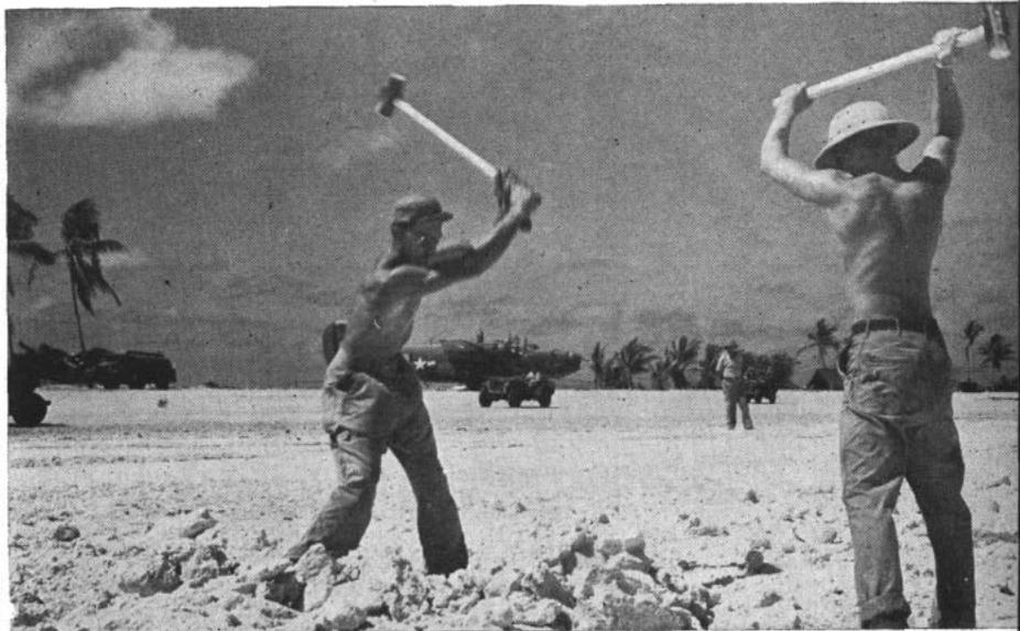
SEABEES attached to Acorns have job of building new airfields and improving and repairing captured fields. Husky Seabees (above) pound coral lumps into sand for Eniwetok runway. Another airstrip (below) is built of metal mats.
