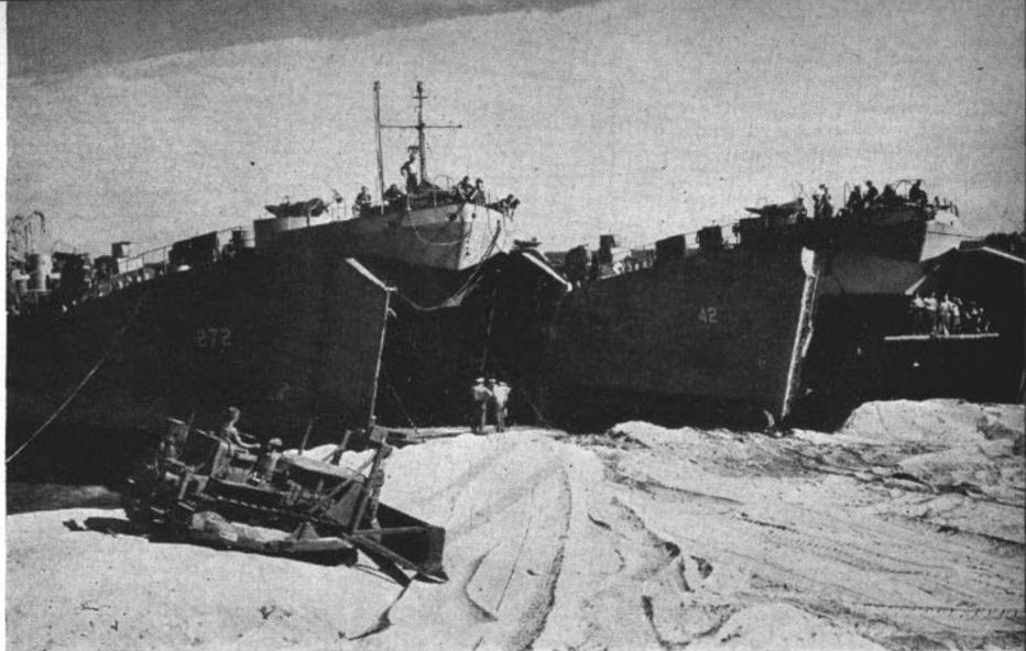
LSTs are generally used by Acorns to move their knocked-down prefabricated airfields to islands in forward areas where there are no docking facilities. Bulldozers, the first gear ashore, plow a causeway to the LST's ramps.
