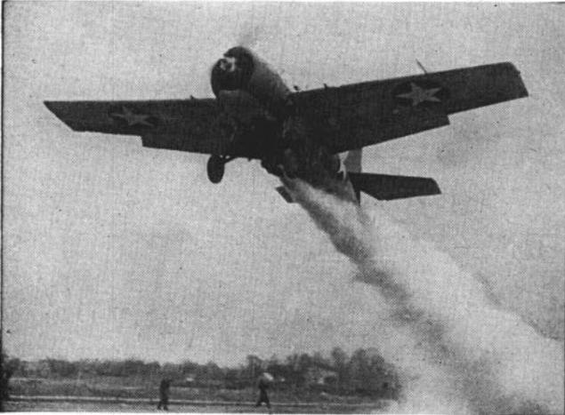
**JATO LEAPS,** or jet-assisted take-offs, reduce take-off runs 33 to 60%, make possible heavier bombloads, use of small airstrips, quick getaway from limited lagoon area or crowded flight deck.
