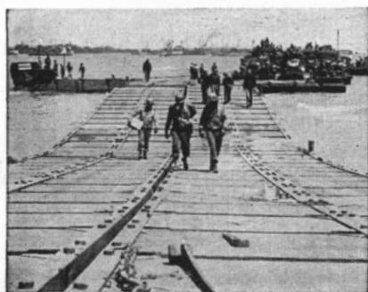
**CAUSEWAY**, one of several, slopes down from beach to floating pier-head for unloading landing craft.
