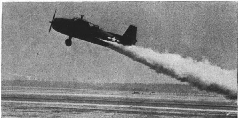
Avenger springs aloft with assistance of four 330-horsepower jet units.
